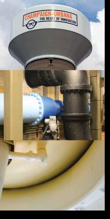
CHAMPAIGN, IL • The interior of the access tube of the Champaign-Urbana CET received two coats of Series 971 Aerolon Acrylic, the innovative, fluid-applied thermal insulating coating ideal for condensation control. The tank utilized several other high-performance Tnemec coatings for its interior and exterior steel and concrete surfaces, too, including Series V700 HydroFlon for extended color and gloss retention.
