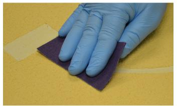
**Step 1:** Identify the area of the coating where corrosion or damage has occurred. Using a utility or sharp putty knife, remove the Series 971 coated surface around the affected area. Lightly sand the edges of the trimmed surface and prepare the substrate according to SSPC-SP 2 or SP 3 Hand or Powering Tool cleaning. Apply the specified primer according to the product data sheet.
