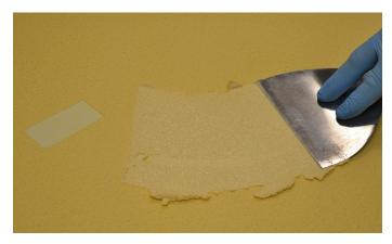
**Step 2:** Once the primed surface has properly cured, use a putty knife to apply Series 971 ensuring the surface is fully covered. Backroll with a loop roller or lightly coat the repaired area with a hopper gun to achieve a consistent appearance with the surrounding coating. Do not exceed 50 mils DFT per lift to avoid cracking due to surface cure. Multiple applications may be required to achieve the original Aerolon thickness.
