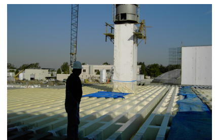
Series 406 Elasto-Shield protects the concrete modules at the Orange County Sanitation District’s secondary treatment facility against biogenic sulfide corrosion.
