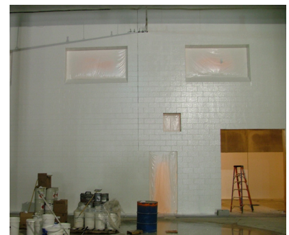
Series 270 Stranlok, a fiberglass-reinforced epoxy coating, protects the walls at Palermo Pizza in Milwaukee, Wisc., from the thermal shock of daily high-pressure steam cleaning.
