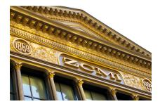
The historic cast iron façade of the ZCMI building in Salt Lake City, Utah, was restored to like-new condition using an advanced fluoropolymer coating system from Tnemec. The façade is now part of the new Macy's department store in the downtown City Creek development. Photos courtesy of Robert A. Baird., Historical Arts & Casting , Inc.
