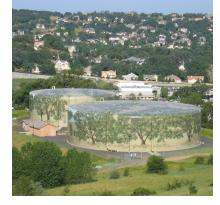
Murals were painted on the Oakridge water tanks in Placerville, Calif., with the same aliphatic acrylic polyurethane coating used as an overcoat on both tanks.
